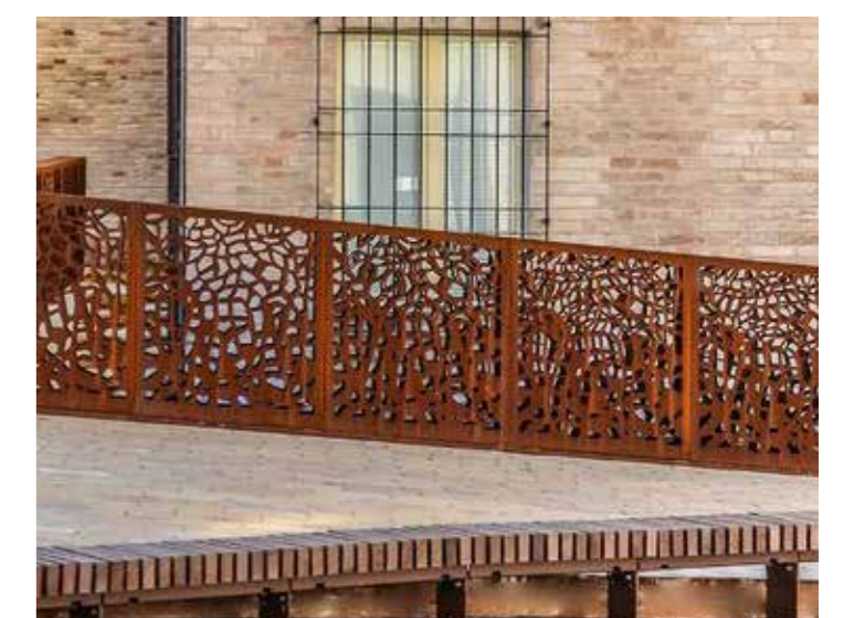
Laser cut corten steel panels can be used as fencing or inset into concrete
